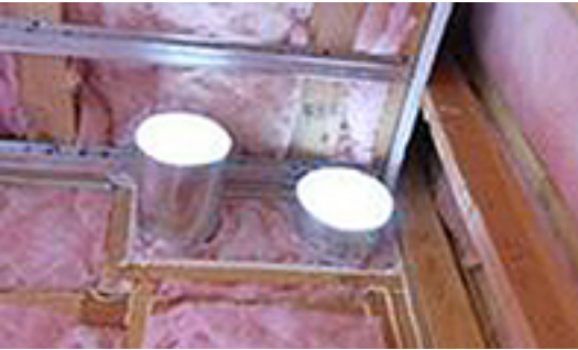
Indoor air is vented to outside rather than into attic.
