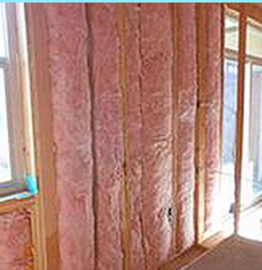
Quality Insulation Installation (QII).
