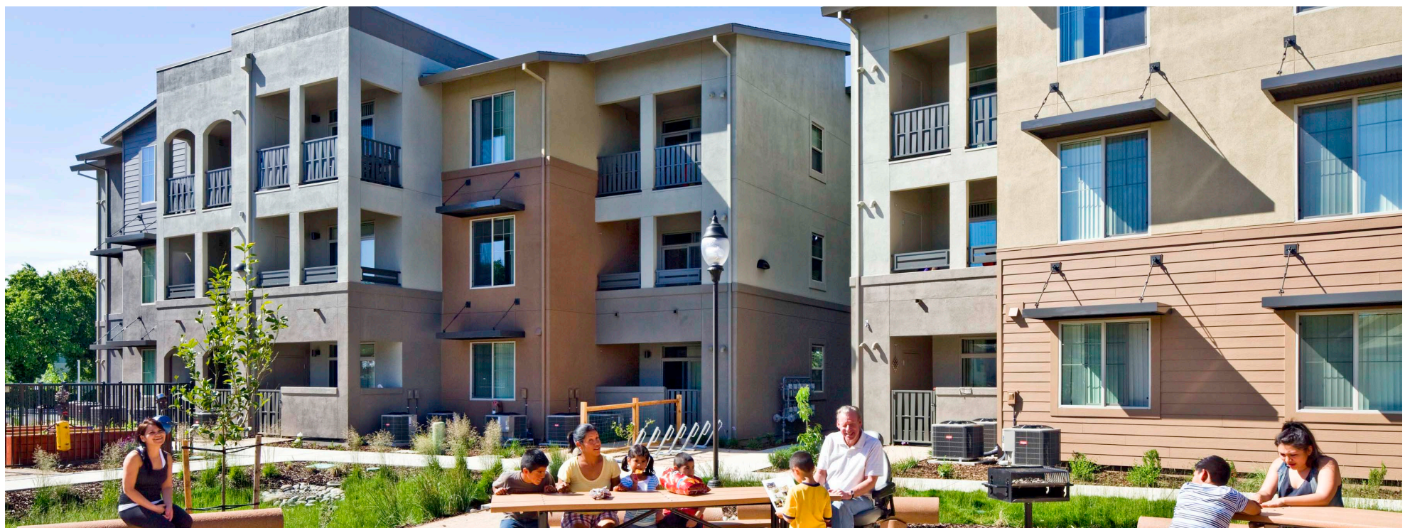
New Harmony Mutual Housing Community, a Davis affordable rental family community
